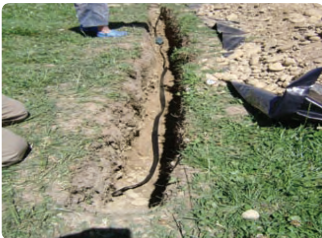
Figure 5. Installing aquaflex
